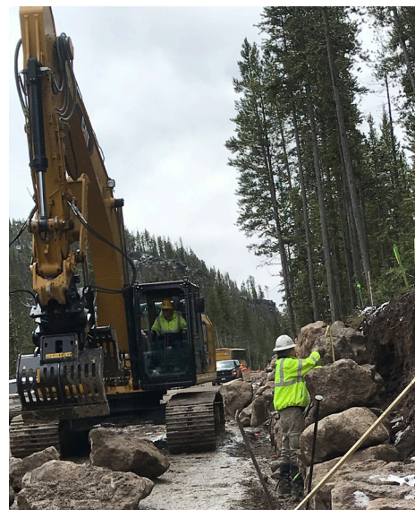
Road repairs in Yellowstone National Park. (Credit: The Pew Charitable Trusts)
